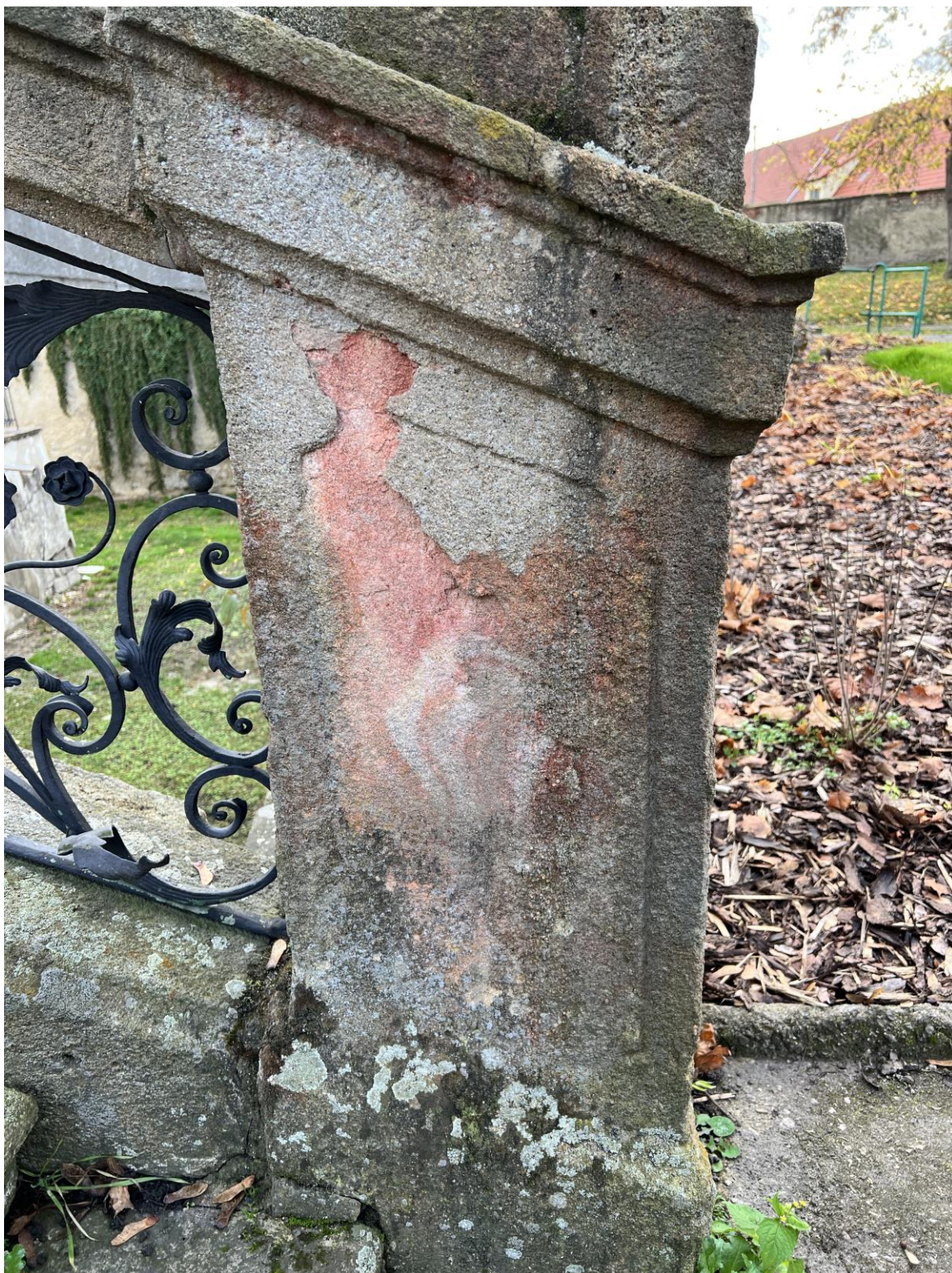
Detail degradace kamene
